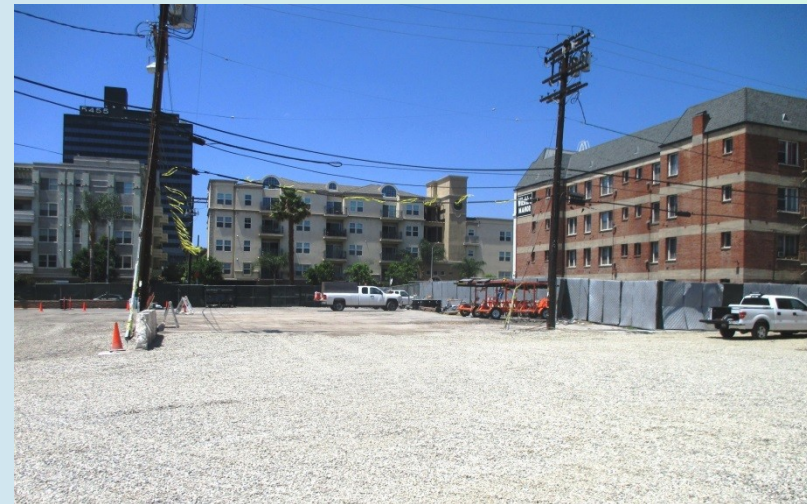
Site Preparation at Wilshire/La Brea North Yard
