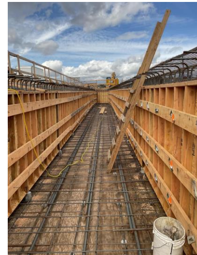
Carpentry work at Butte Canyon Bridge
