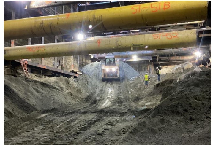
Century City Constellation Station - Excavation Progress
