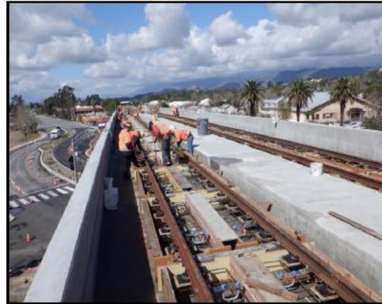
Bonita / Cataract – Structure Track Direct fixation
