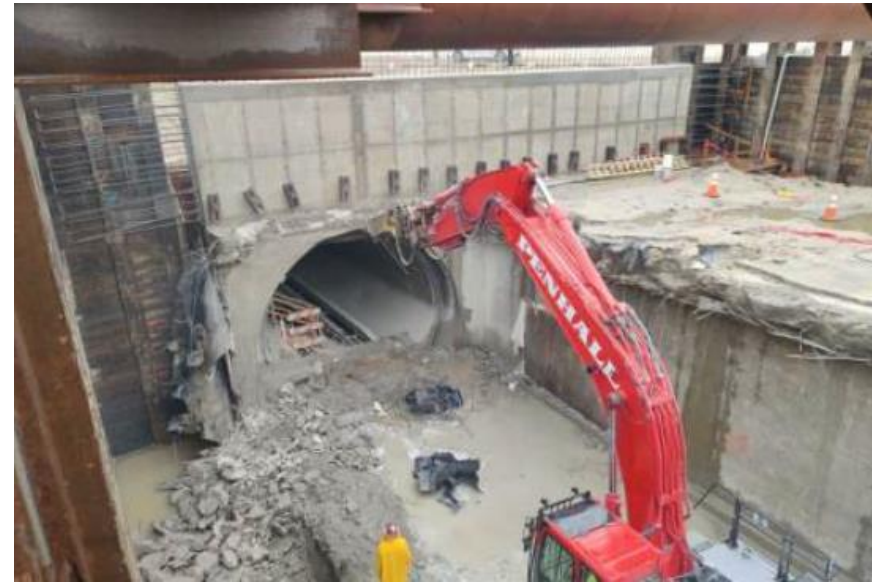
West Portal Wall Demolition
