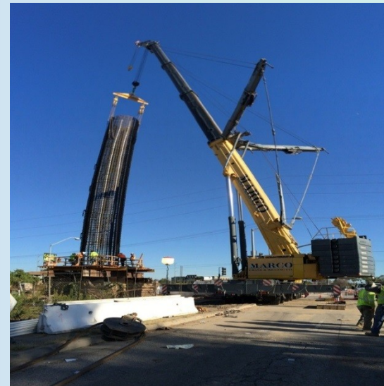
I-405 BRIDGE – Bent 2 cast-in- drilled-hole column cage placement
