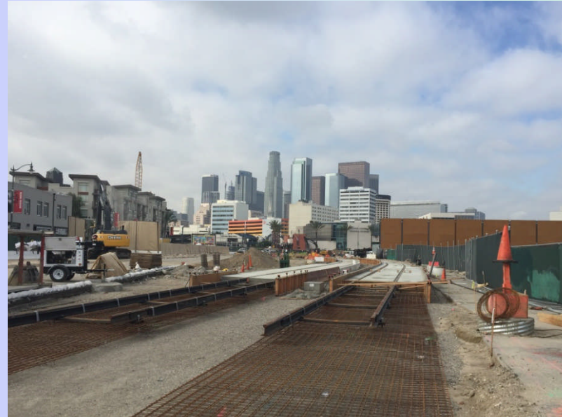
Shoofly installation at Mangrove Yard
