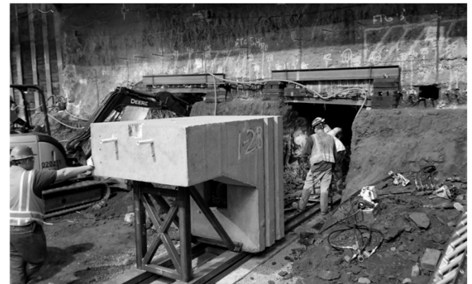
Underpinning activities underway at Historic Broadway Station
