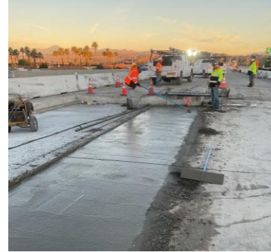
Placement of Lean Concrete Base (LCB) in the median
