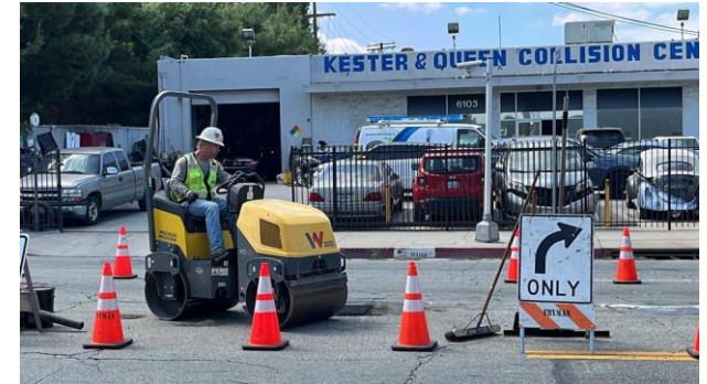
Potholing Restoration on Bessemer St.
