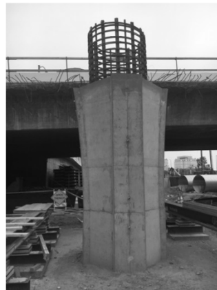
Completed bridge column
