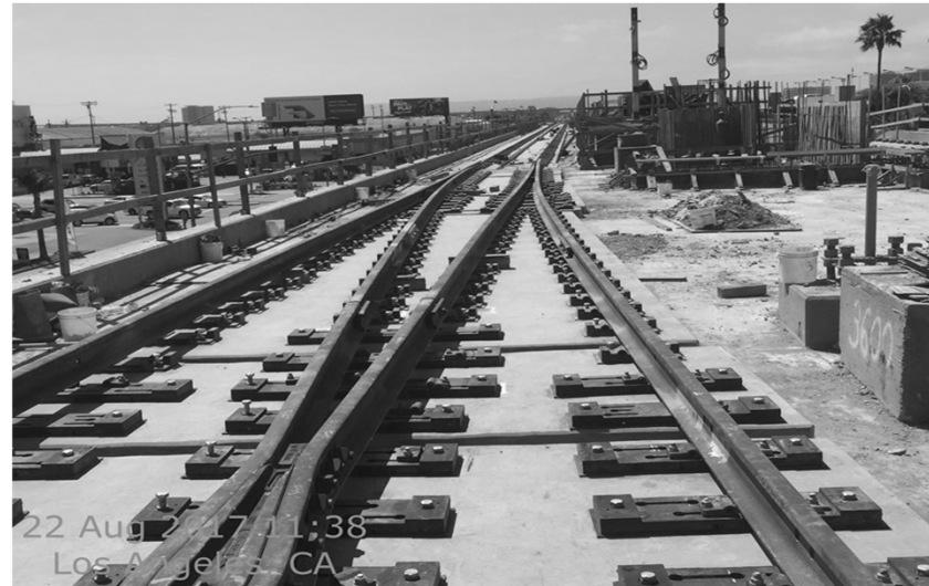
Switch for crossover at Aviation/Century Bridge.
