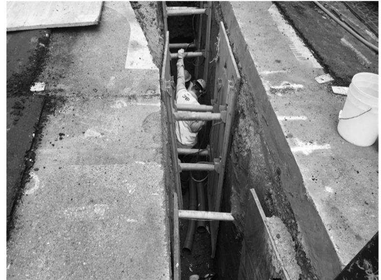
LADWP power relocation work in Century City
