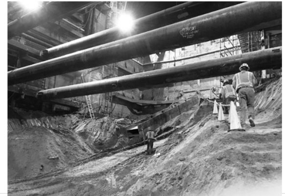
Under Deck Excavation at Wilshire/La Brea Station
