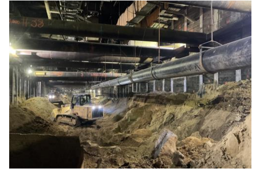
Century City Constellation Station Box Excavation
