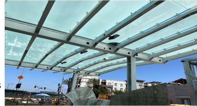
Plaza Canopy at Little Tokyo/Arts District Station
