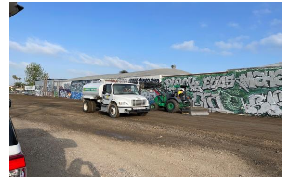
Site preparation work
