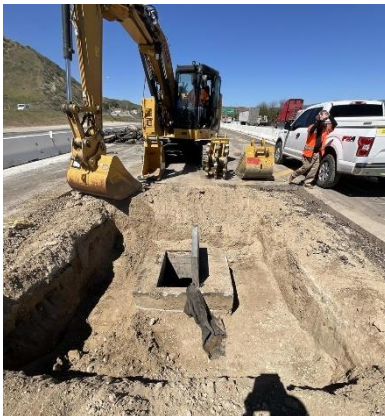
Stage 1 Phase 1 Drainage Inlet Installations in Median
