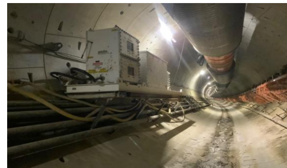
BL Tunnel Booster Fan & Transformer Installation
