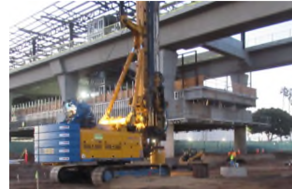
CIDH pile work near APM Station
