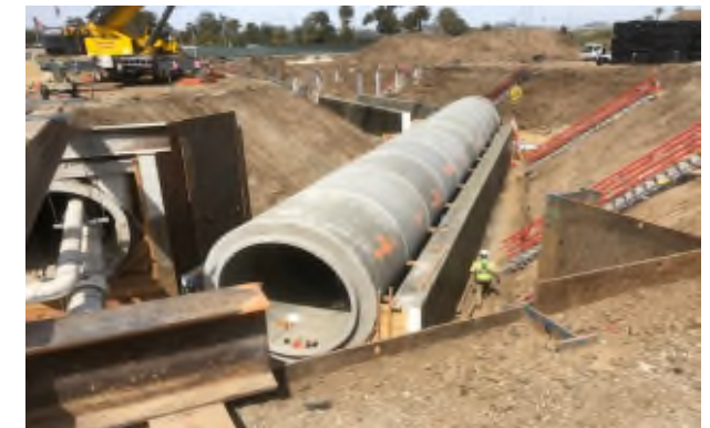
Installation of Steam Tunnel RCP in Concrete Cradle
