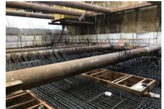
Rebar Installation at Wilshire/Rodeo Station Entrance
