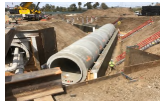
Installation of Steam Tunnel RCP in Concrete Cradle
