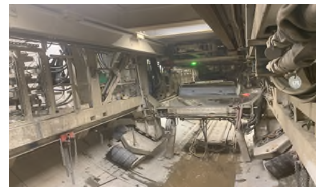
BR TBM Ring Segment Installation
