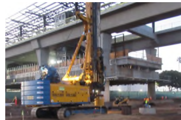
CIDH pile work near APM Station
