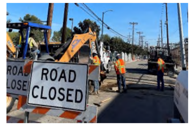
DWP Sylmar Undergrounding
