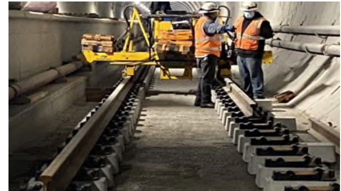
Track Installation in the Reach 1 Tunnel
