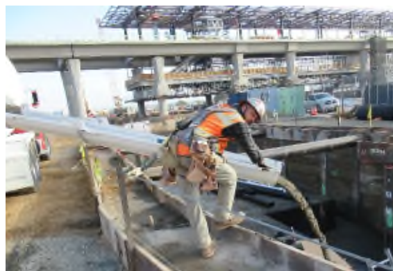
Backfill at cisterns
