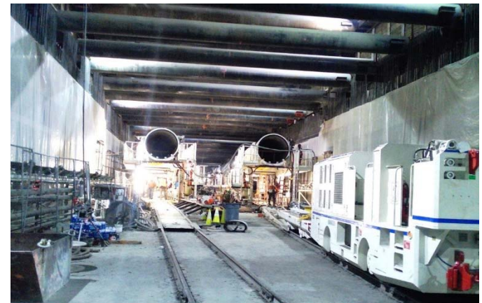
TBM at Wilshire/La Brea Station
