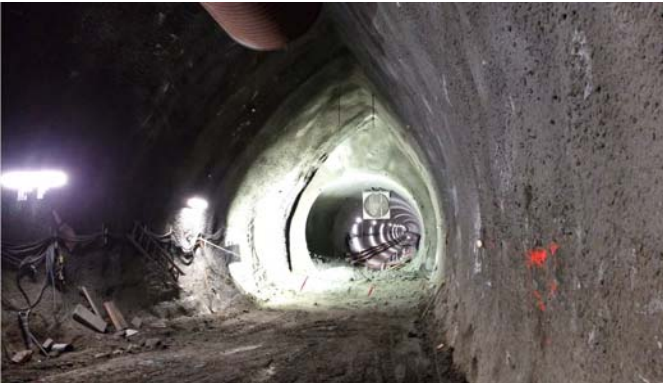
Cross-over Cavern excavation
