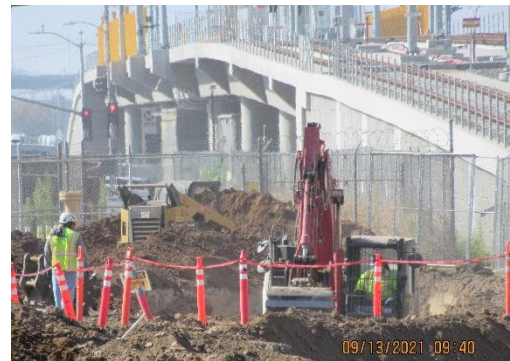
Backfill Work at South End of Site
