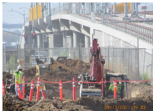
Backfill Work at South End of Site
