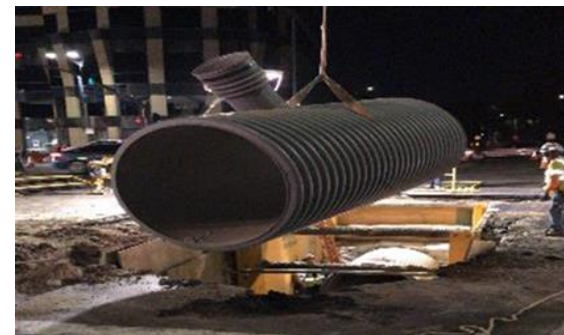
Sewer Relocation for Westwood/UCLA Station
