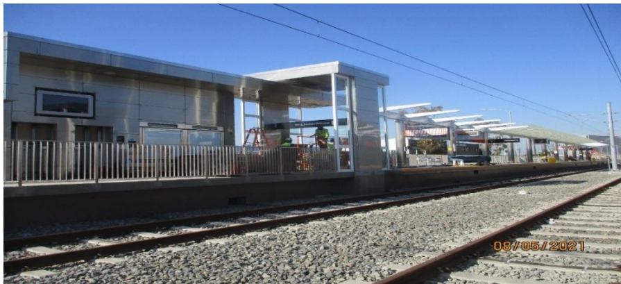
Hindry Station – Mounting wind screen glass
