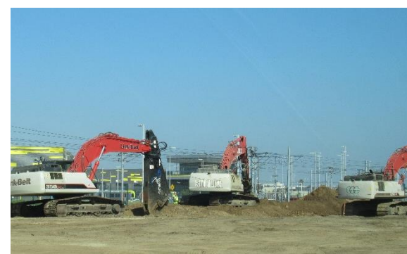
On Site Grading and Backfilling Work
