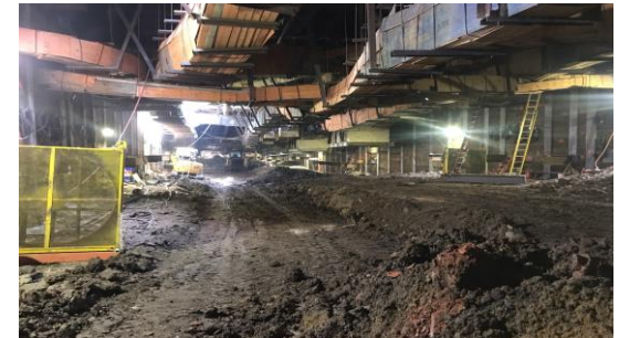
Constellation Station Box Excavation
