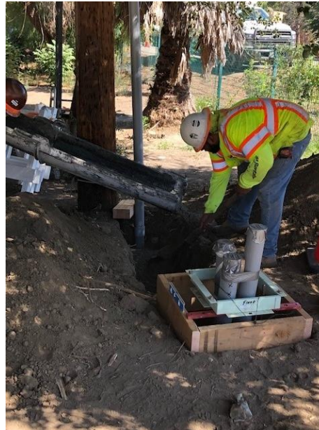
Pilot Gate - DWP Service Pedestal Installation
