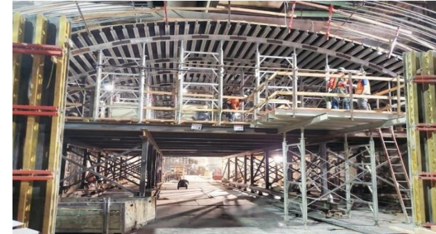
Roof Falsework Installation at Wilshire/Fairfax Station
