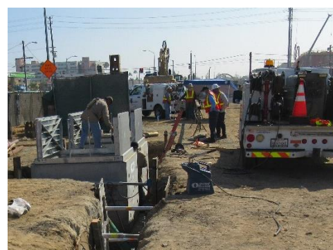
Utility Work on Arbor Vitae
