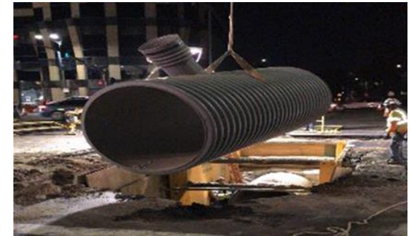
Sewer Relocation for Westwood/UCLA Station
