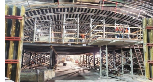
Roof Falsework Installation at Wilshire/Fairfax Station
