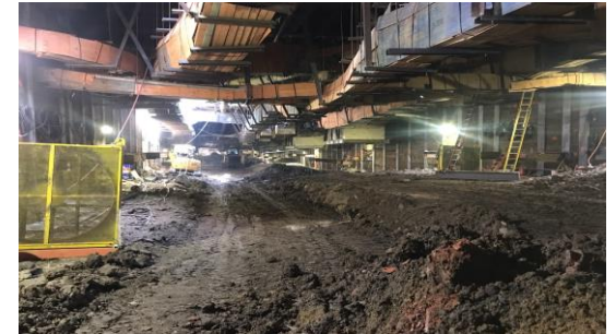
Constellation Station Box Excavation
