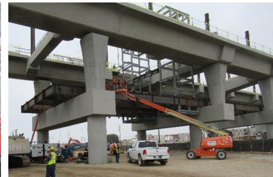
LAVA APM Steel Work in Progress
