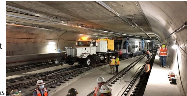
Dead pull test in Crossover Cavern
