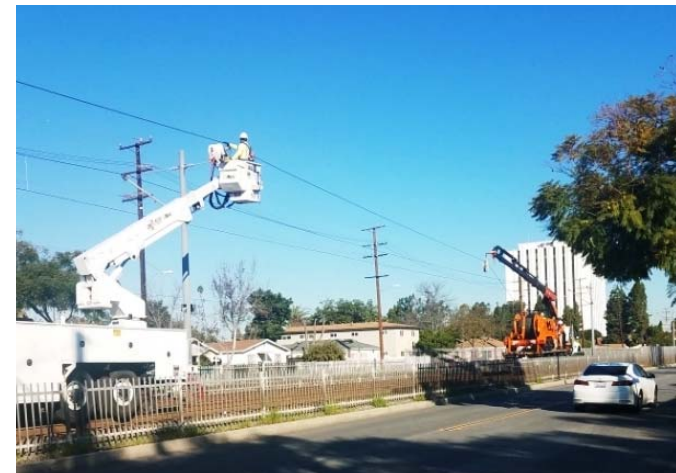
Overhead Catenary System Demolition
