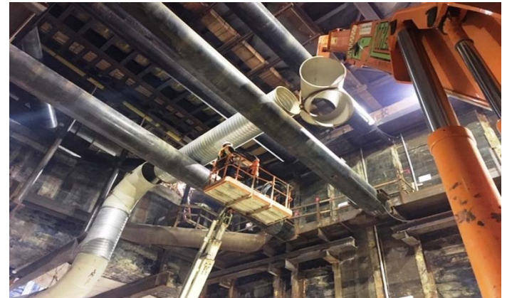
Reconfiguration of Ventilation at the Western Shaft
