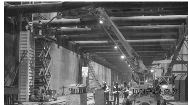
Concrete placement for columns in Expo Station
