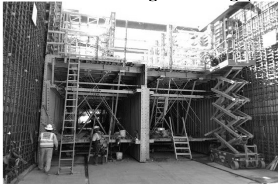
Concrete wall construction continues in UG1
