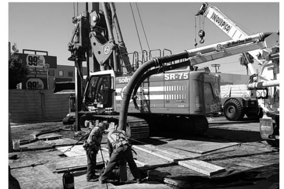
Pile installation activities at Wilshire/Fairfax Station
