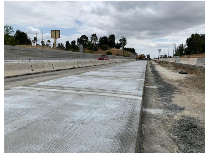
Stage 2 Median Paving Joined Plane Concrete Pavement.
