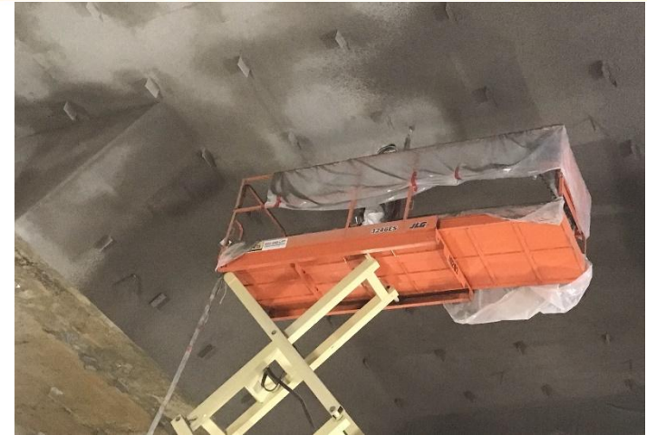
Century City Station Acoustical Treatment on Ceiling
