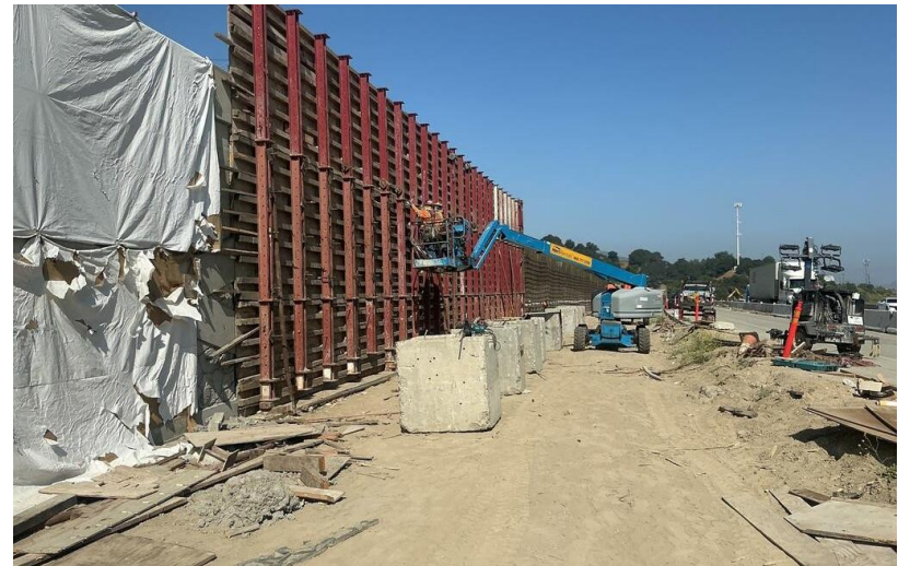
Retaining Wall 2449 Formwork Installation
