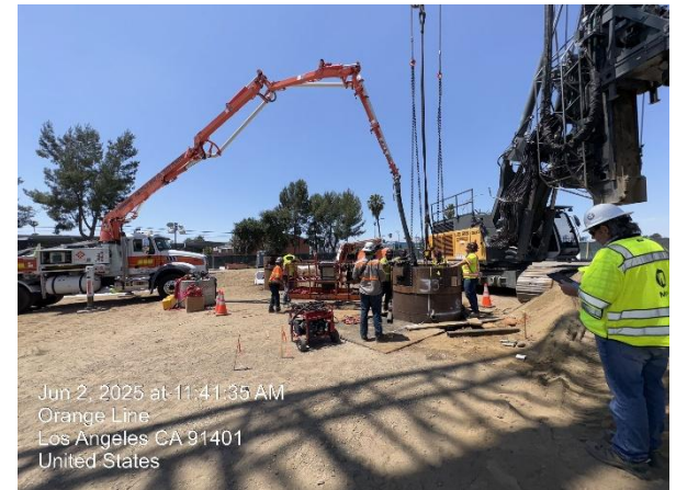
CIDH Foundation Installation at Van Nuys
