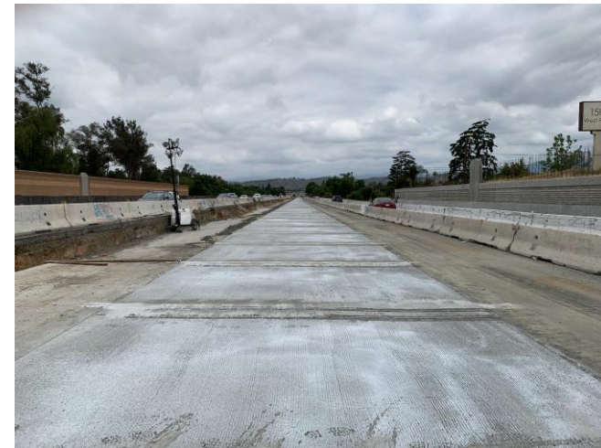
Stage 2 Median Paving Joined Plane Concrete Pavement.
