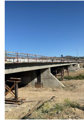
Castaic Creek Bridge Falsework Lowering
