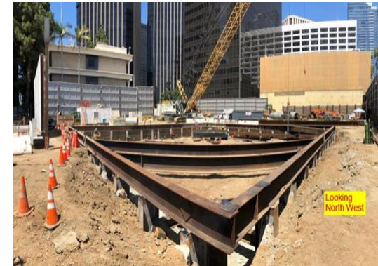
Tunnel Shaft Excavation in Century City
