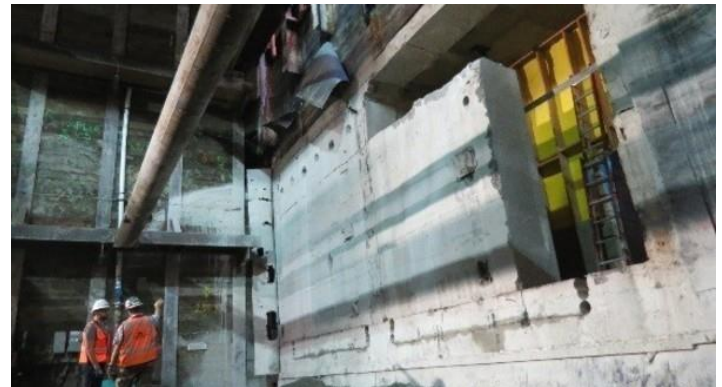
Break through knock-out panel at 7 th /Metro Center Station
