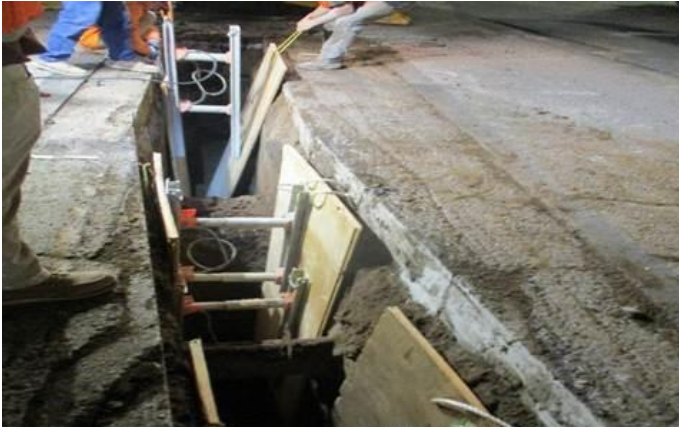
Hand Dug Excavation for Fiber Optic Conduit
