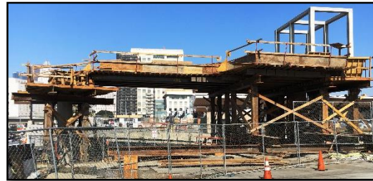
Elevator Platform Falsework
