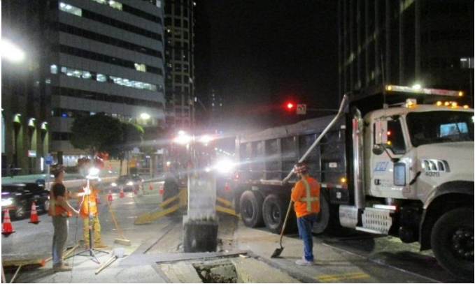
Main Line A Excavation and Potholing
