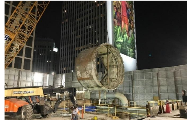
TBM Gantry Shield at Wilshire/Western
