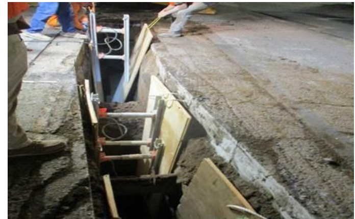
Hand Dug Excavation for Fiber Optic Conduit
