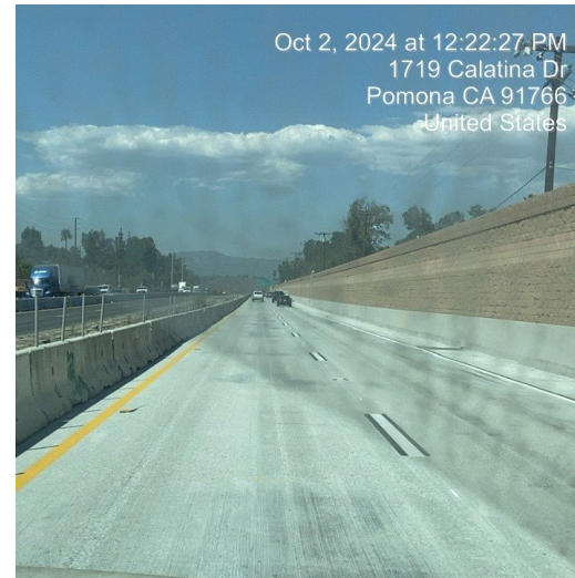
NB-71, completed stage 1 roadway.
