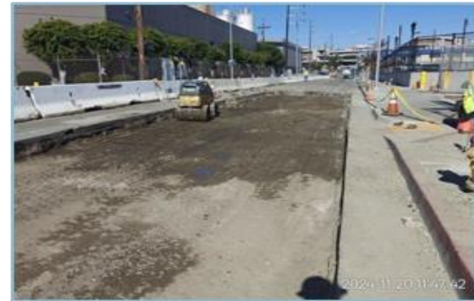
Center Street Reconstruction
