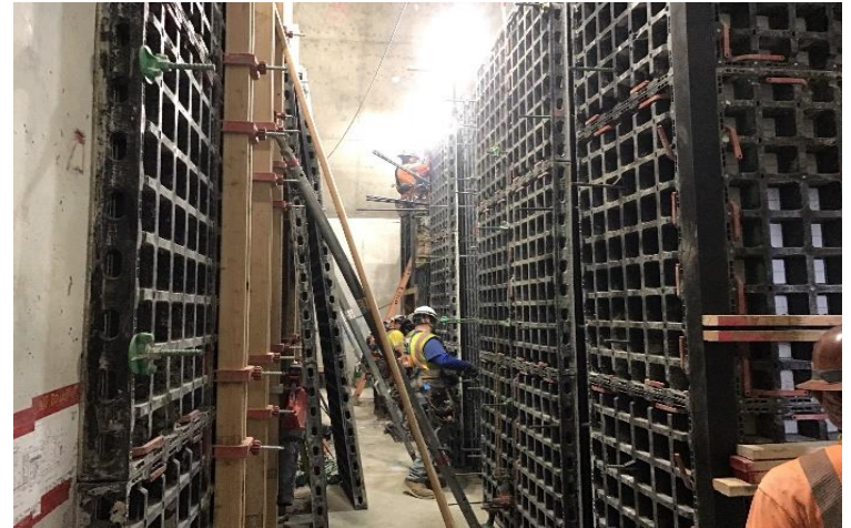
Wilshire Rodeo Station Interior Walls-East Concourse Level Slab
