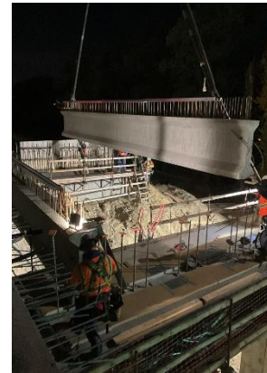
Set Girders at Rye Canyon Bridge
