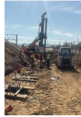
Wall 986 Installation of 24IN CIDH Piling
