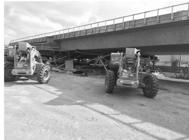
Aviation Station/Century Bridge – removing forms
