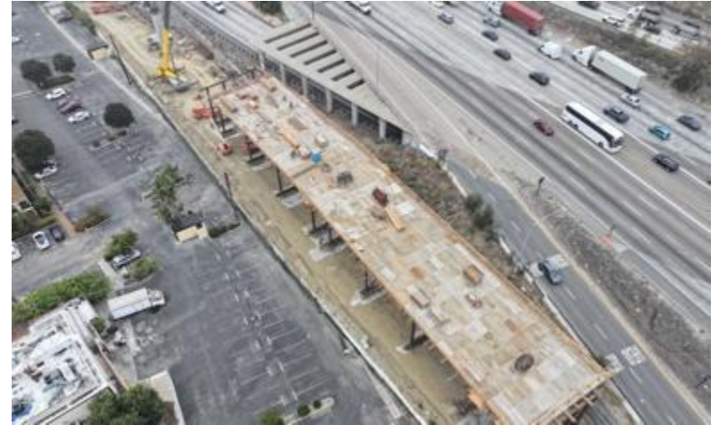
Falsework for EB SR-60 Bypass Bridge Deck
