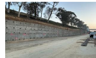
105WB RW 270 Soil Nail Wall Exterior
