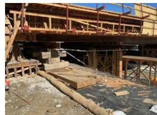
105EB Stanford bridge falsework
