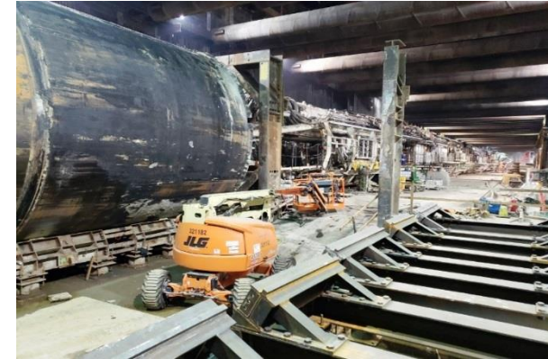
Purple TBM at Wilshire/Fairfax Station
