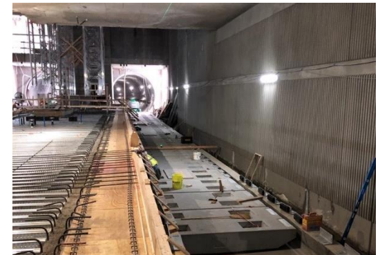
Pre-cast Floating Slab at Grand Av Arts/Bunker Hill Station
