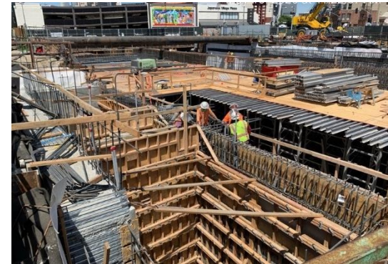
Interior wall installation at the future Little Tokyo/Arts District Station
