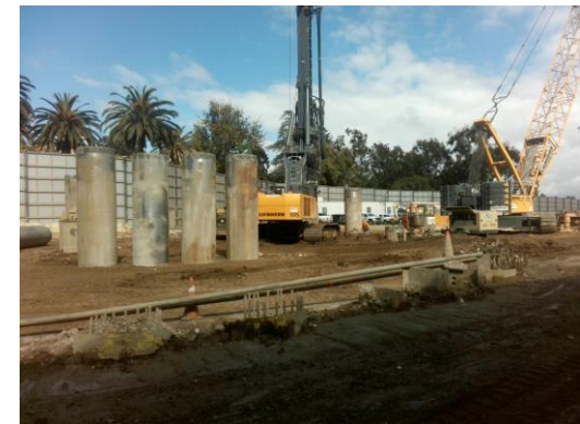
Pile Installation for TTES
