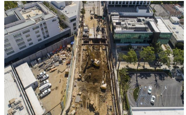
Street Decking Installation on Wilshire Boulevard
