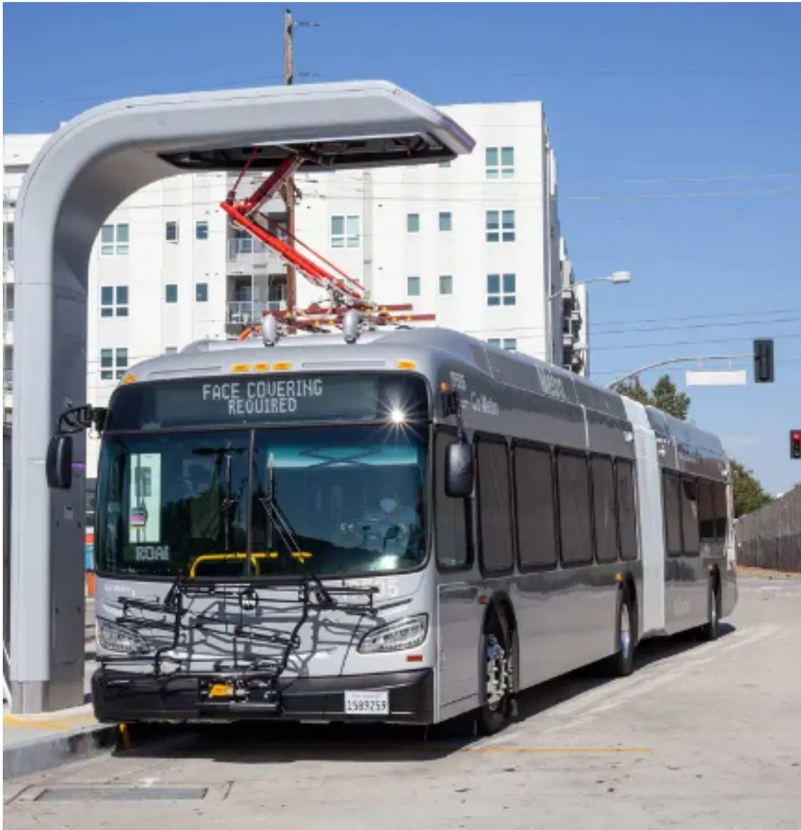
Figure E.2-1. North Hollywood Station On-Route Charger
