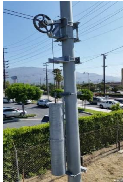
Figure 15: Existing weight stack tensioning system
