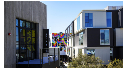
Figure 19 Platform, a transit oriented development in Culver City adjacent to the Expo Line, is a carefully curated retail experience with restaurant and creative office space.
