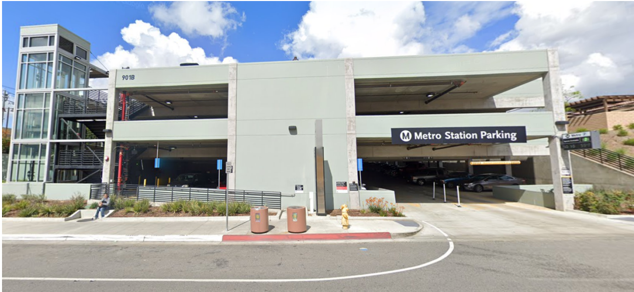
Figure 4.10.4 APU/Citrus College Parking Garage (view from Citrus Avenue)
