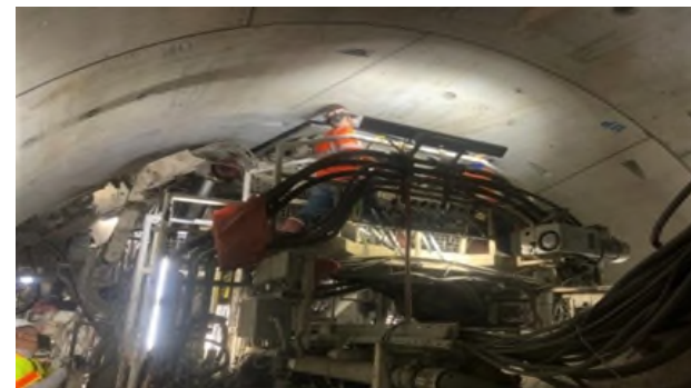
Ring Installation in the BL Tunnel
