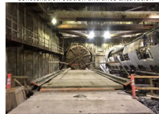
Ruth Breakthrough at Wilshire/Rodeo Station
