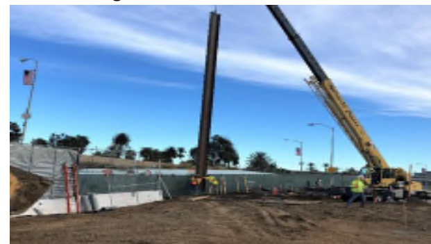
SOE Pile Installation for VA Steam Tunnel Relocation
