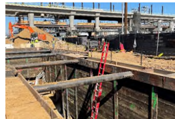
Shoring near completion for east cistern
