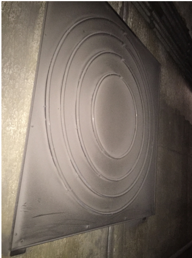
Metro Blue/Expo Tunnel – Outdated electrical artworks not functioning as intended
