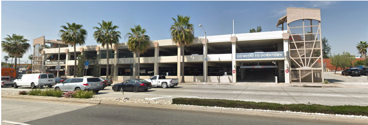
Figure 4.10.2 Atlantic Parking Garage (view from Atlantic Boulevard)
