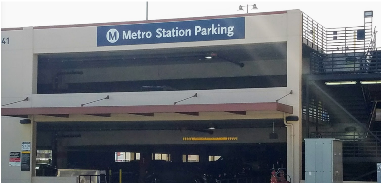
Figure 4.10.7 Monrovia Parking Garage (view from Primrose Avenue)
