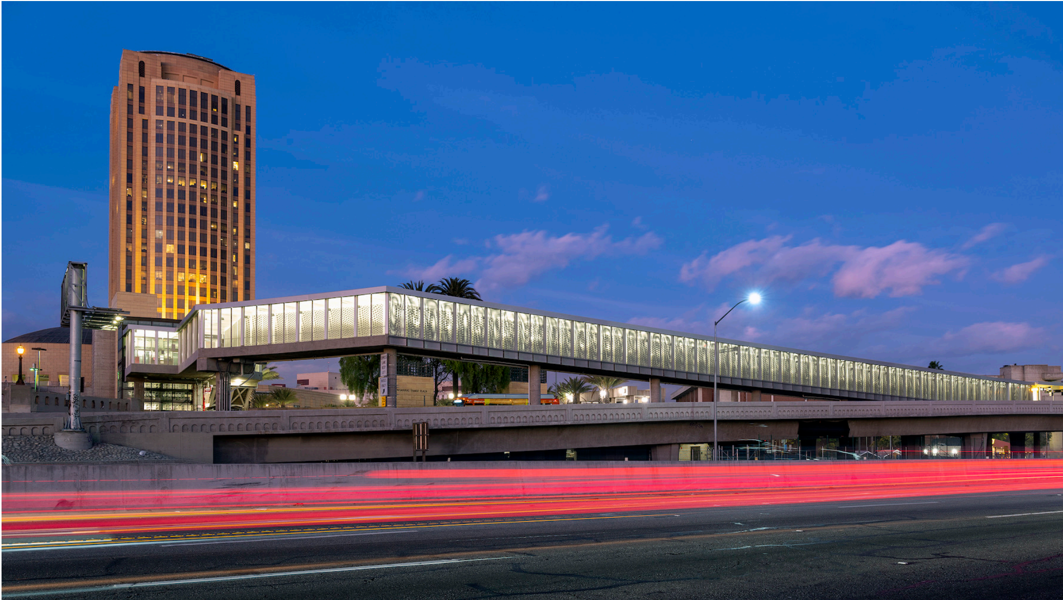
Ned Kahn | Wind Bridge | Patsaouras Plaza Bus Station
