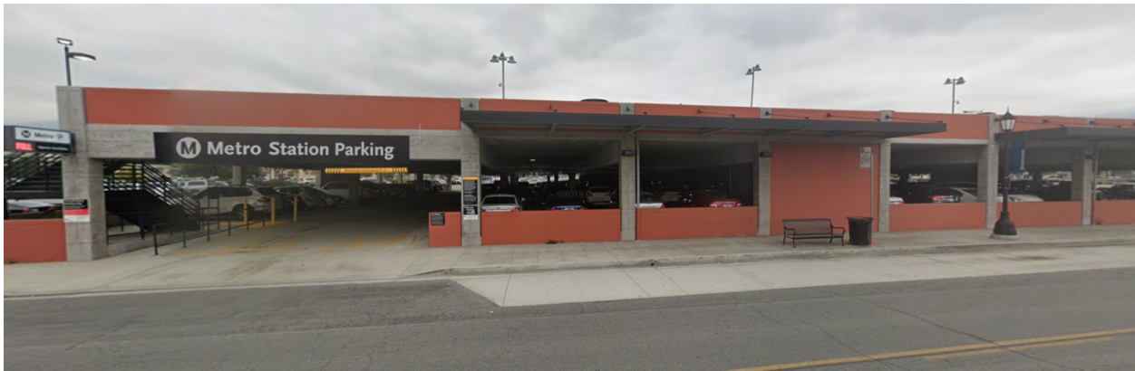
Figure 4.10.5 Arcadia Parking Garage (view from Santa Clara Street)
