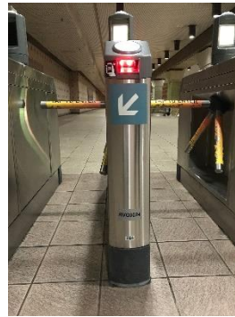
367 Gates 154 Emergency Gates
