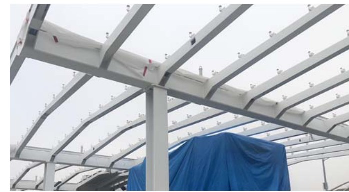
Little Tokyo/Arts District Station Canopy Installation
