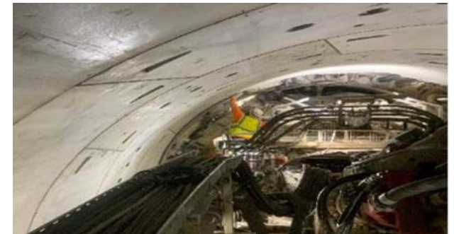
Ring Installation in the BL Tunnel
