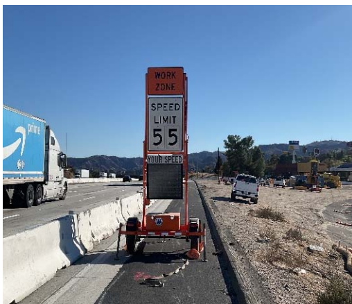
Placement of temporary work zone speed radar and stormwater pollution prevention materials
