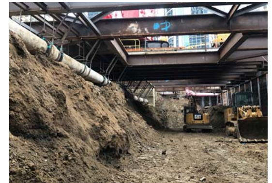
Constellation Station Entrance Excavation
