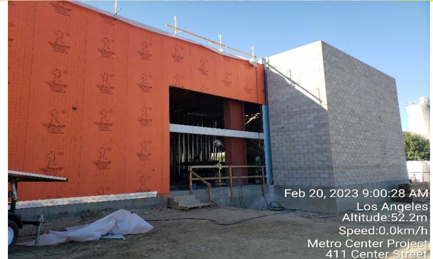
Exterior Finish – Weather Barrier & Sheet Metal
