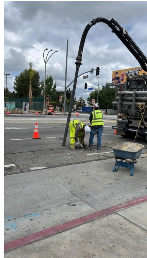
Potholing at Van Nuys Blvd
