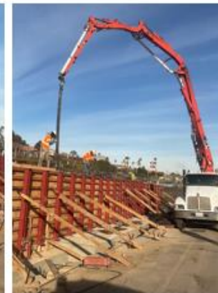
Forming, preparations, and concrete pour at Retaining Wall 2622
