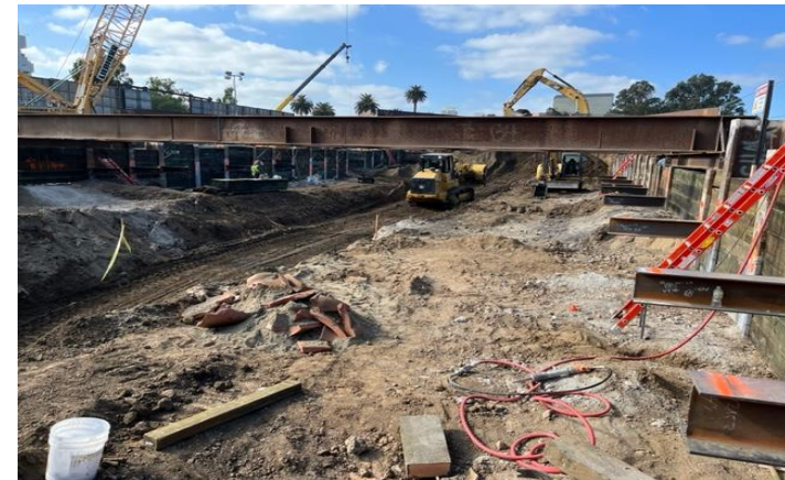
Westwood/VA Station: Excavating station to Level 1 Bracing
