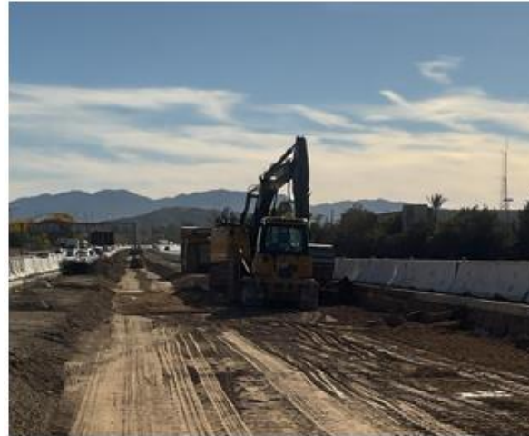
On-Going Roadway Excavation in the Median
