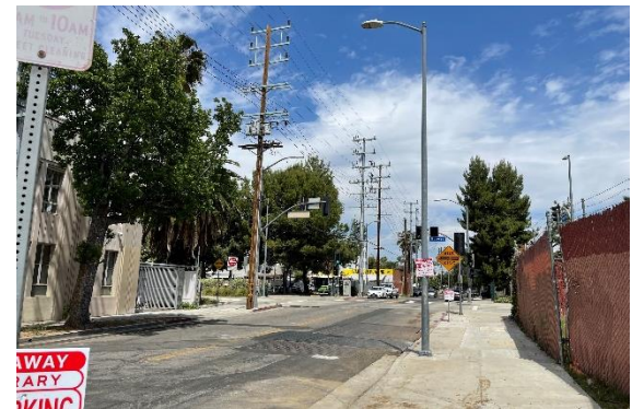
DWP Overhead Construction at Vesper
