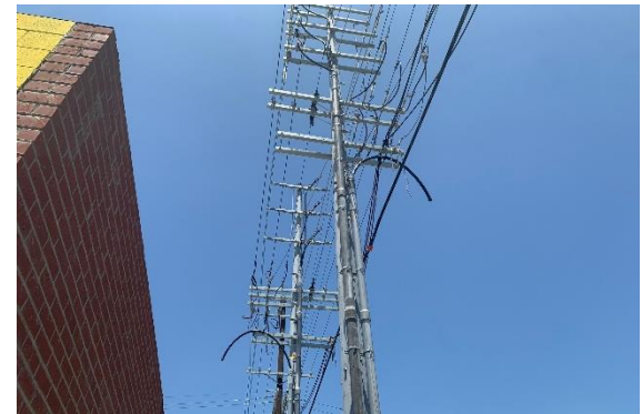
DWP Overhead Construction at Vesper
