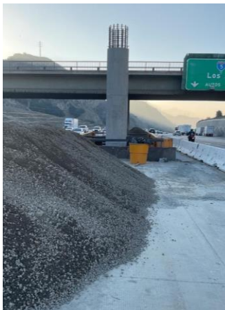
Erection of Column for new Weldon Canyon bridge
