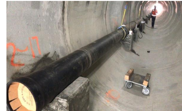
Westwood/VA – VA Steam Tunnel Relocation Installation of 12-in Ductile Iron Waterline
