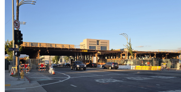
Falsework for Van Nuys Bridge
