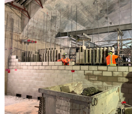
Westwood/VA Hospital Station: Upper Interior Masonry Wall Construction
