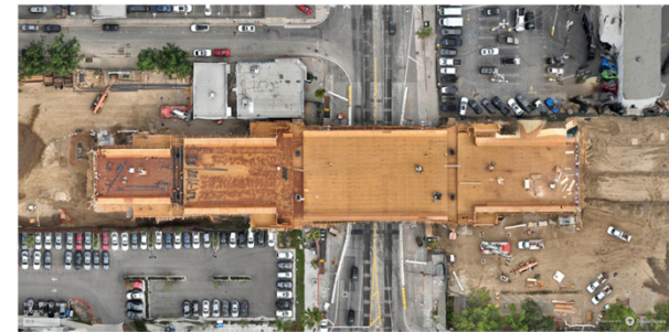
Aerial View of Van Nuys Bridge Construction
