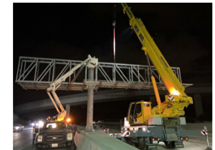
Sign Structure Truss Installation
