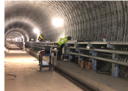
Tunnels: Steel Walkway Construction BL Tunnel
