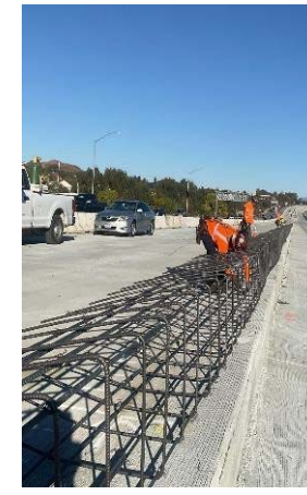
Median Barrier Rebar Installation
