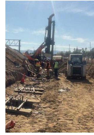
Wall 986 Installation of 24IN CIDH Piling
