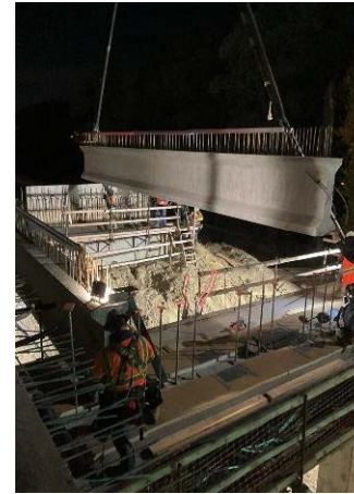
Set Girders at Rye Canyon Bridge
