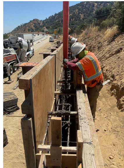
Pouring concrete at Retaining Wall 2461
