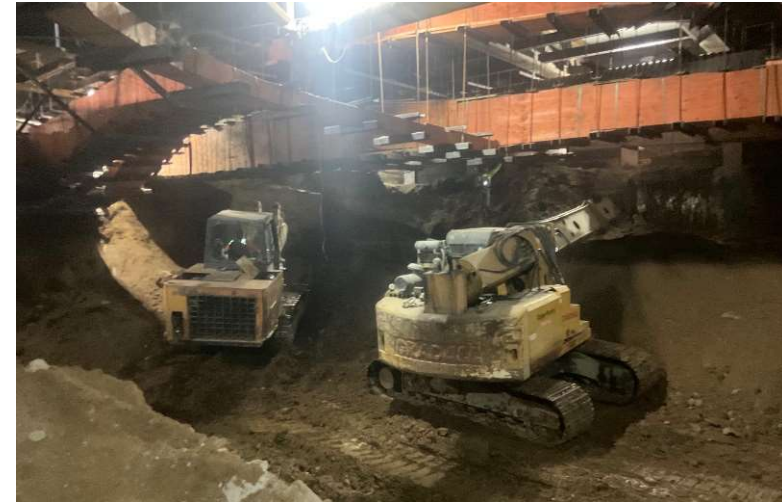
Westwood/UCLA Station: Excavation at Wilshire Blvd
