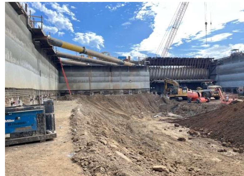
Westwood/VA Station: Tiebacks & Shotcrete Installation and Excavation
