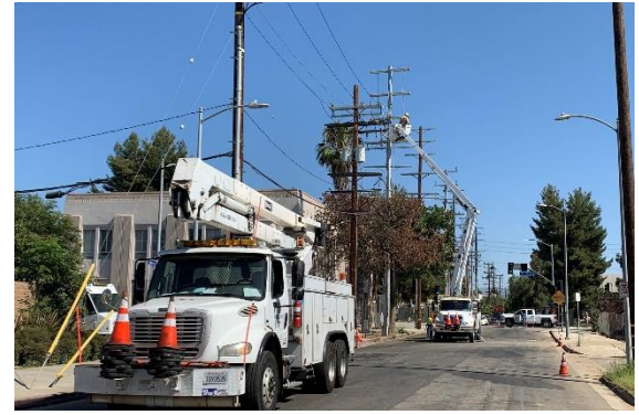
DWP Overhead Construction at Vesper
