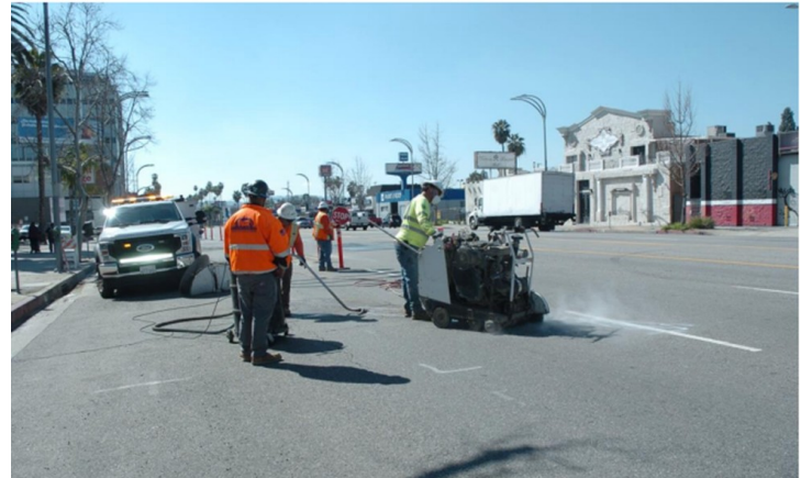
W.A. Rasic crew saw cutting pavement on Van Nuys Blvd. near Hartland St.
