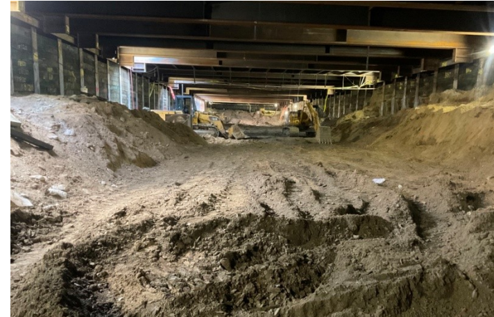
Westwood/UCLA Station: Excavation underneath Wilshire Blvd
