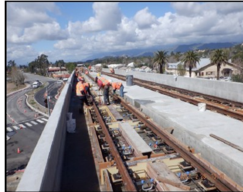
Bonita / Cataract – Structure Track Direct fixation
