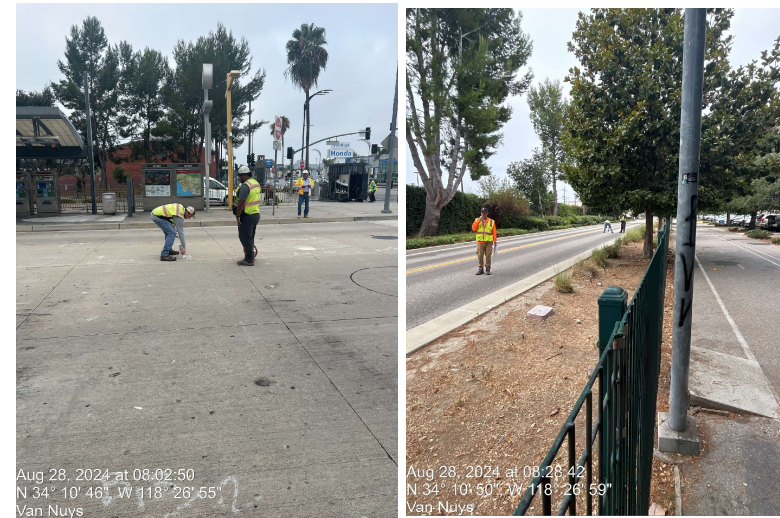
Phase II Environmental Site Assessment – Site Walk & Soil Boring Marking at Van Nuys
