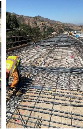
Gavin Canyon Bridge Deck Rebar Install
