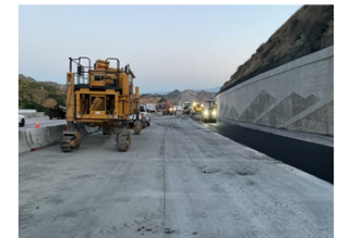
AC Paving NB Gavin Canyon
