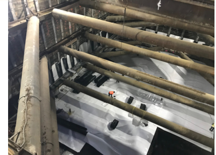
Westwood/UCLA Station: Completed Northeast Entrance Excavation and Waterproofing Installation
