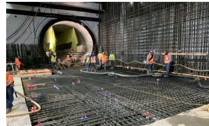
Concrete Placement at Wilshire/La Cienega Station (West)
