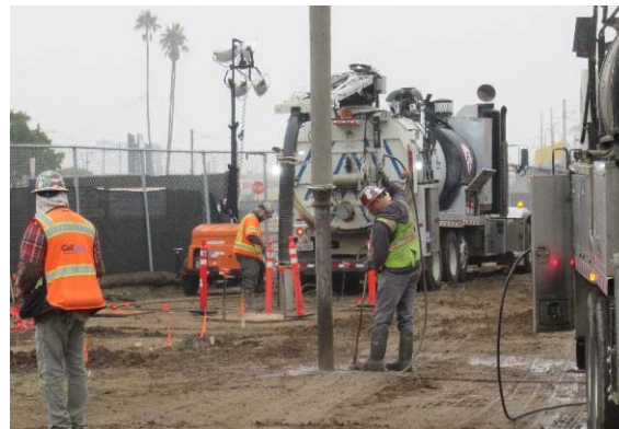
Shoring installation for Stormwater System
