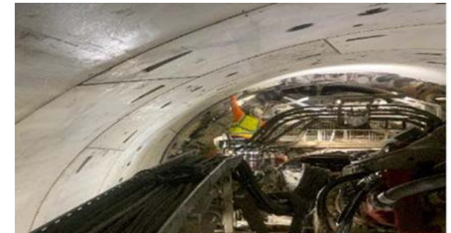
Ring Installation in the BL Tunnel
