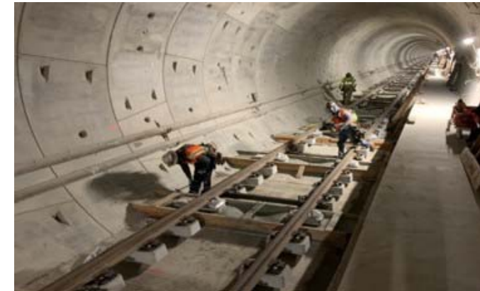
Reach 1 North Tunnel Trackwork Installation
