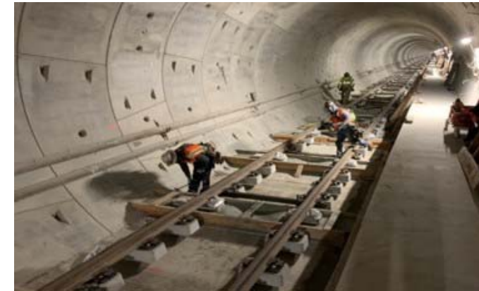
Reach 1 North Tunnel Trackwork Installation
