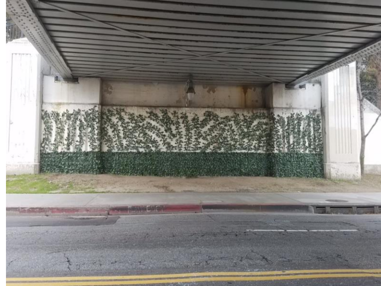
Lincoln/Cypress Station - After
