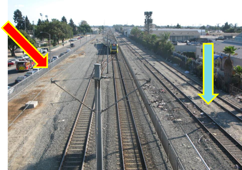
Metro Fence Line & UP Wilmington Sub-Division
