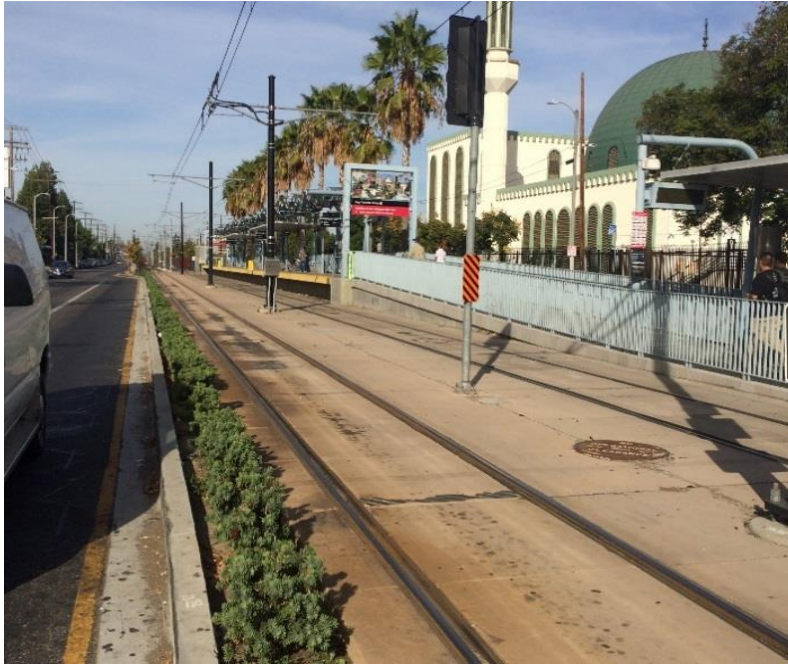
Expo - Expo/Vermont Station – Trash Free
