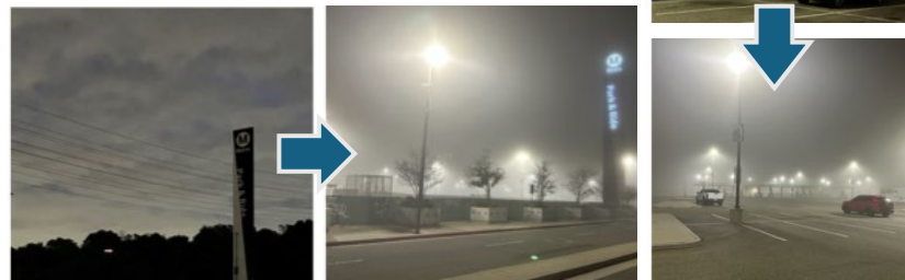
Lighting improvements at Harbor Gateway Transit Center(Before & After)
