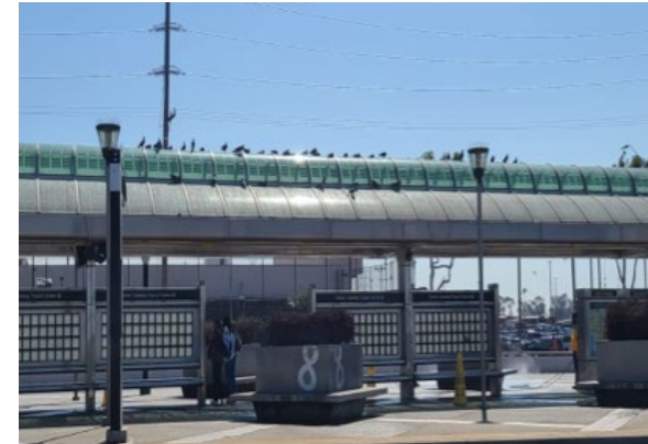
West Canopy – No device installed
