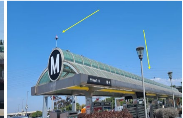
East Canopy – Device INSTALLED
