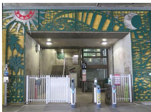
Allen Station After
