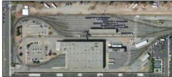
Photo ES-5: Typical LRT MSF Facility and Inside the Main Building
