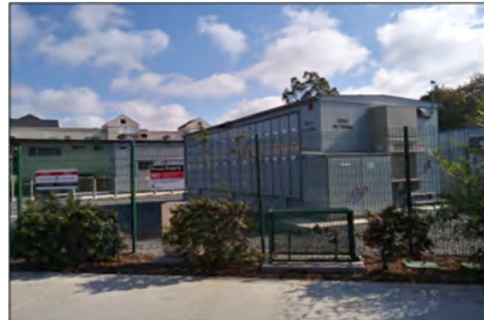
Photo ES-7: Typical TPSS for LRT
