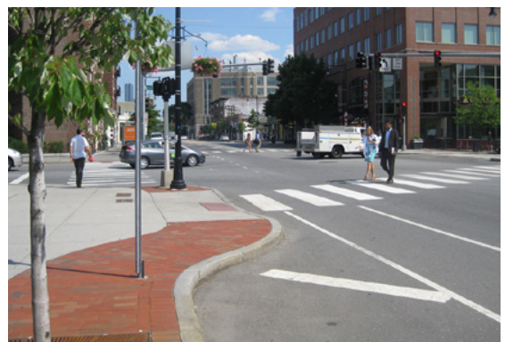
Curb extension and crosswalk
