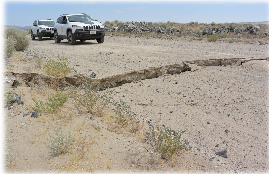
Caption: Fault rupture crosses dirt road, with California Geological Survey vehicles for scale. Displacement at this location is primarily normal (vertical). Photograph taken near the northern end of the rupture resulting from the M7.1 Searles Valley earthquake.
