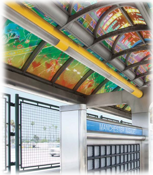
Caption: Manchester Avenue Metro Station
