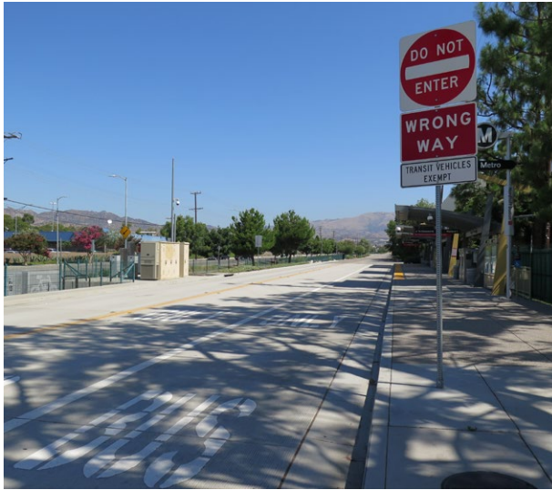
Figure 14. Exclusive BRT roadway
