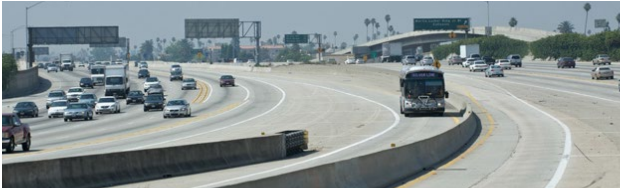
Figure 11. BRT managed lanes
