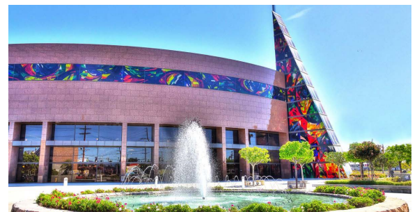
The West Angeles Cathedral is a major destination adjacent to the station.
