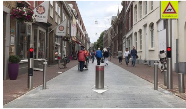
Shared street space with access control in Europe (examples exist where local access or bus is allowed) / Photo Credit: ITVHub
